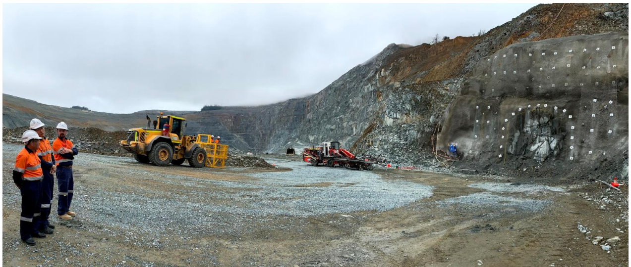
Figure 3 Exploration Decline at the south end of North Pit
