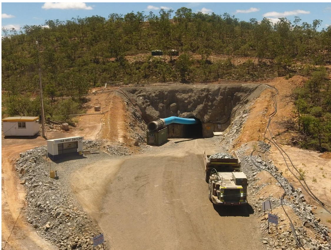
Figure 2 Truck Leaving Far West Decline
