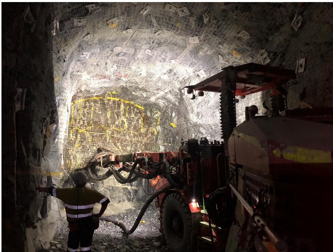
Figure 3 Drill Jumbo at Far West Decline Face
