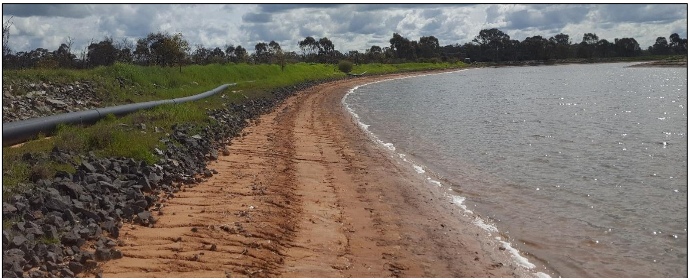
Bund walls screen the ponds with vegetation on the sides.
