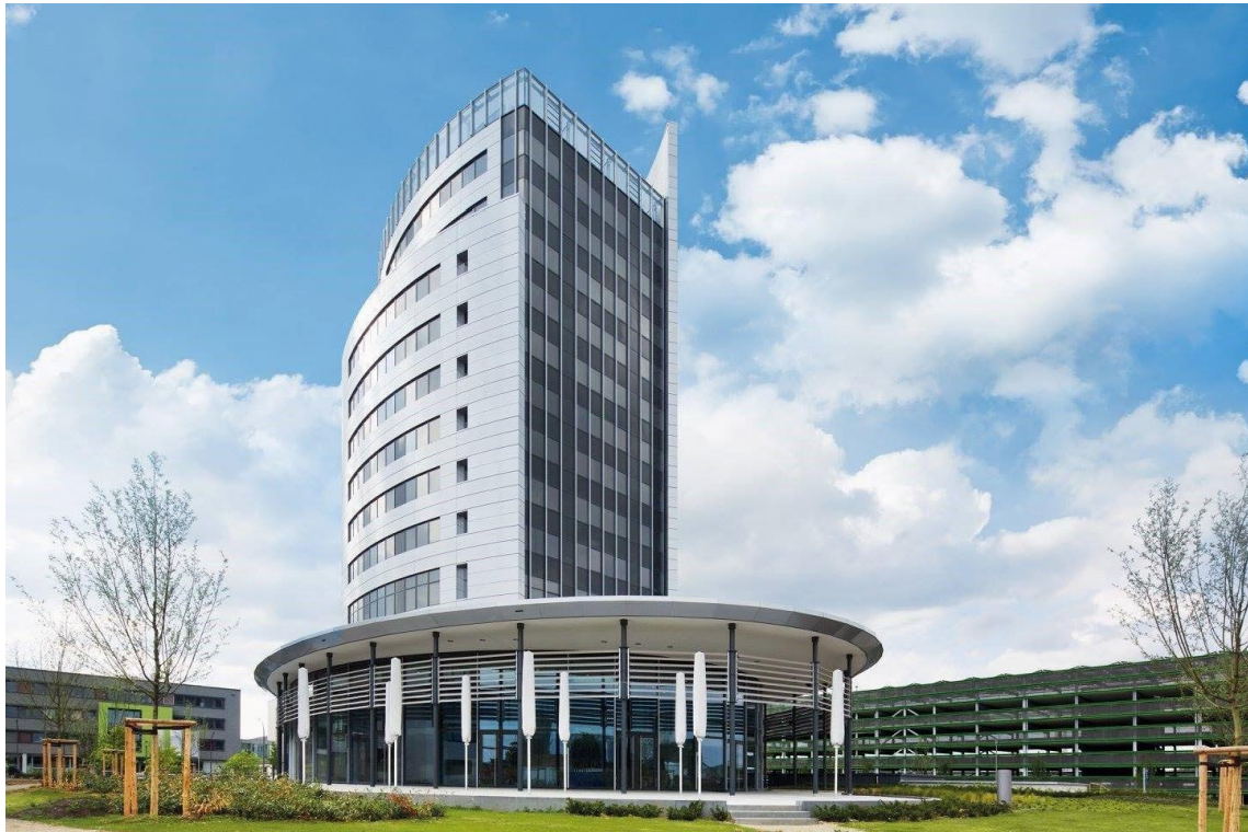
Figure 8: Building in Heilbronn where dataglobal's office is located
