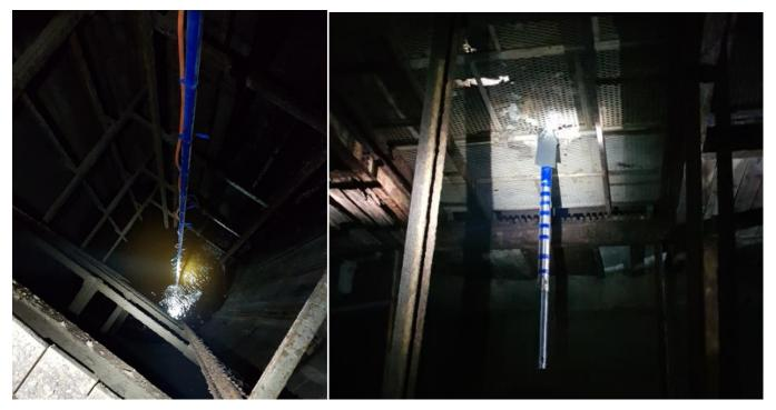
Figure 4: (LHS) Boreline 400 flexible-hose suspended in the Hutchings Shaft, with a 378m vertical lift. This is the longest, single-lift pumping setup using self-supporting flexible hose under trial in the world. (RHS) The 18.5kW Vansan submersible bore pump being lowered in the Hutchings Shaft.
