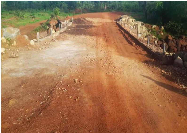
**Makabingui road, culvert masonry works completed**
