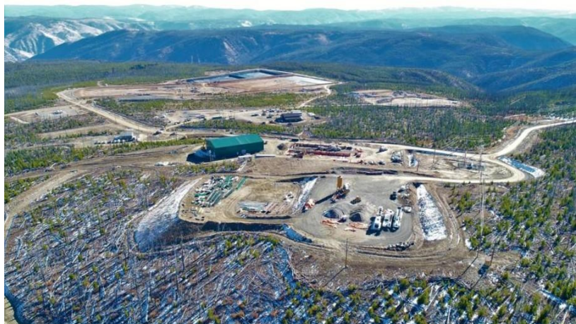
Figure 1 - Jervois' Idaho Cobalt Operations near Salmon, Idaho
