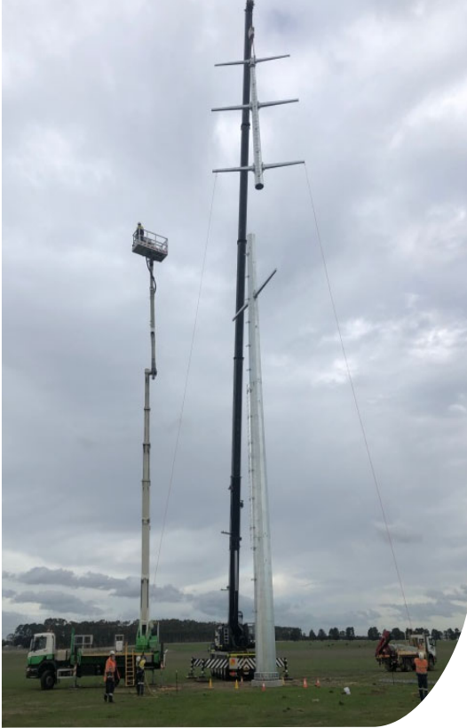
Transmission line pole construction
