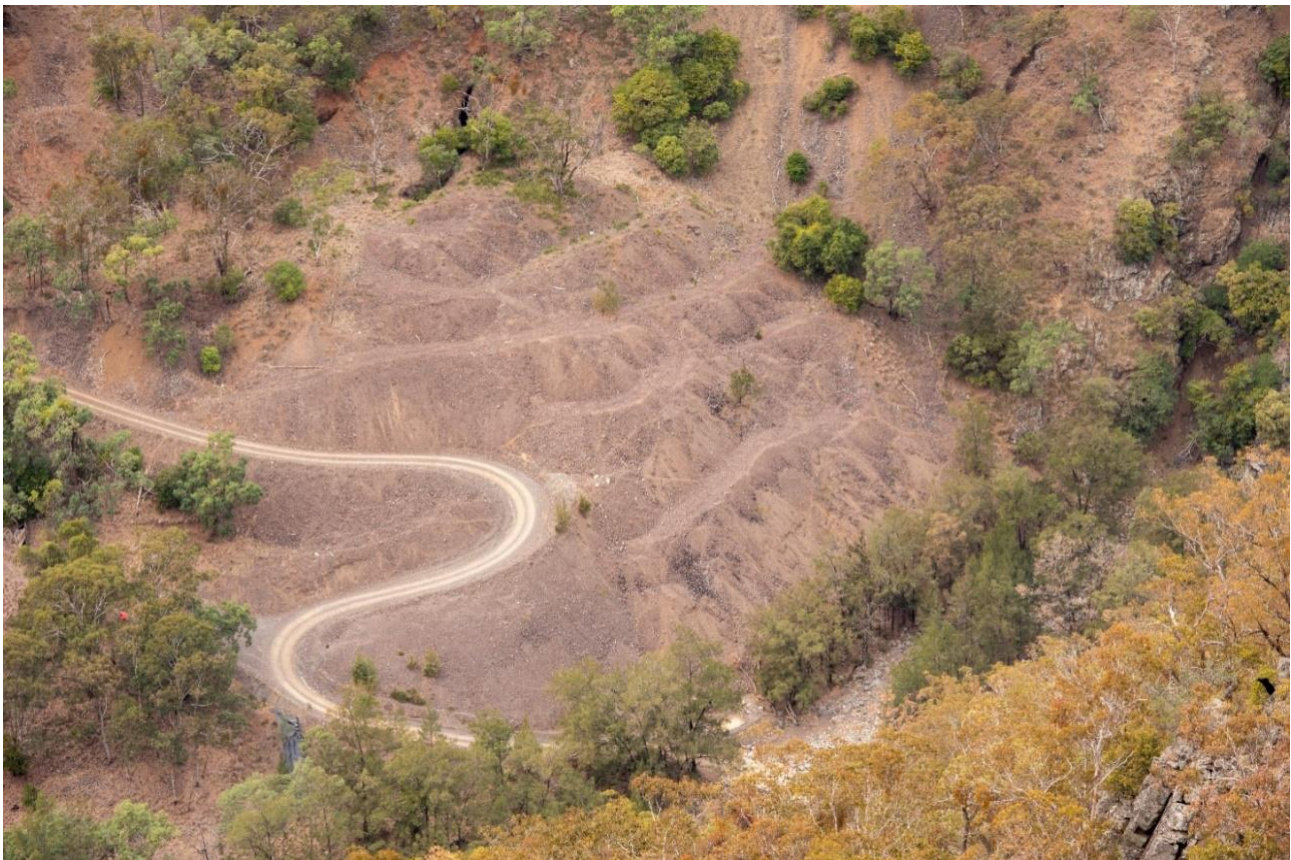
Figure 1 Bakers Creek Waste Rock Dump (August 2019)
