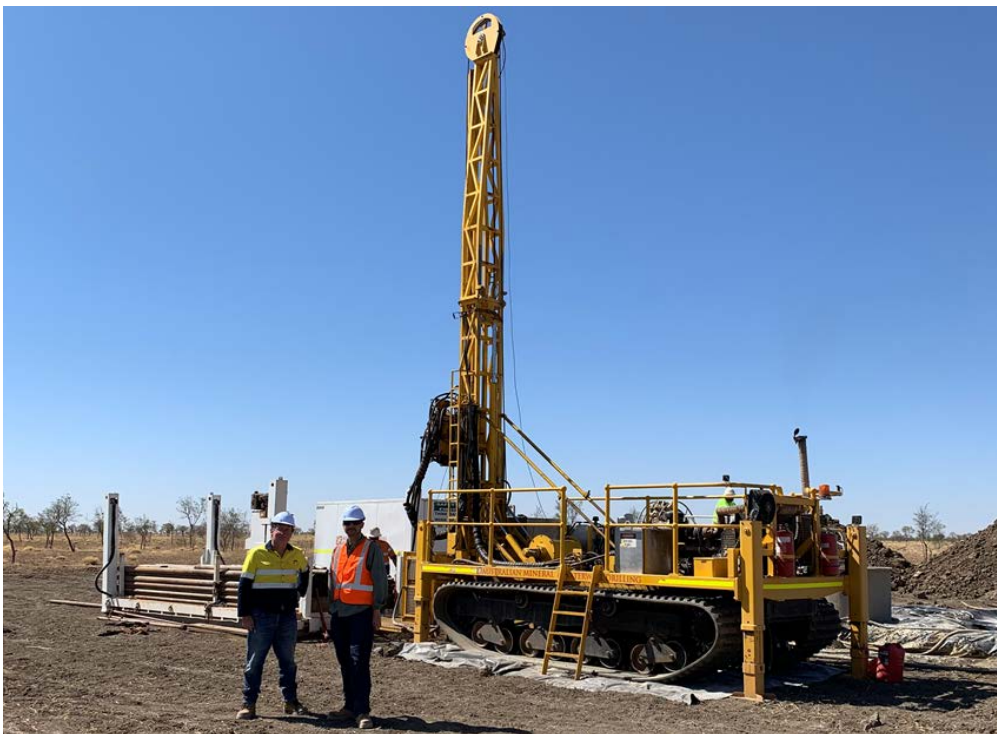
Figure 1: Alton HD900 track-mounted drill rig on site at Saxby
