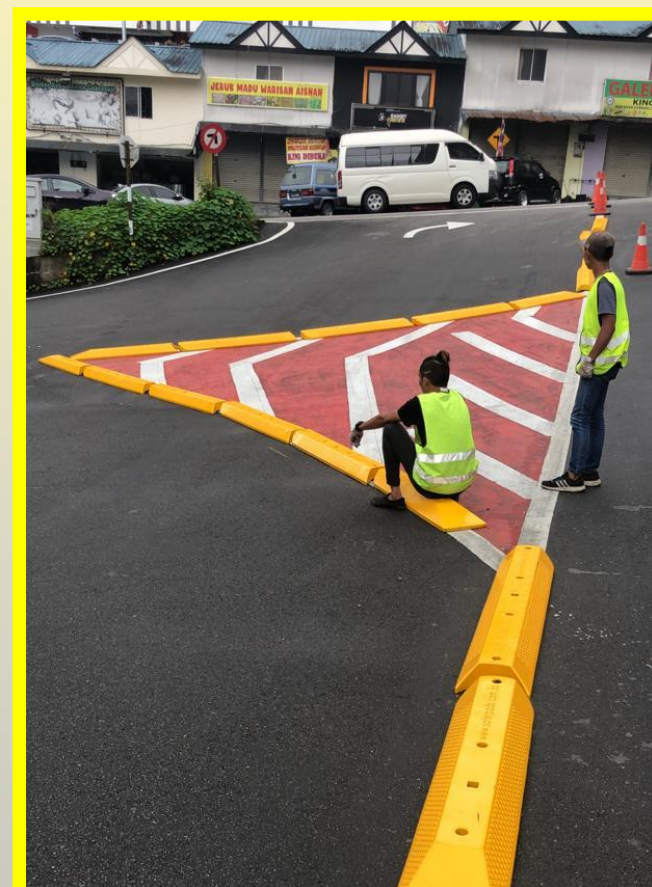
Separation Kerb in Malaysia
