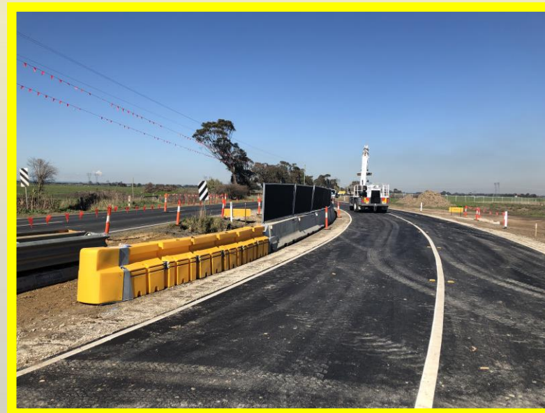
TLOK barriers with screens Road Safety Rental deployment
