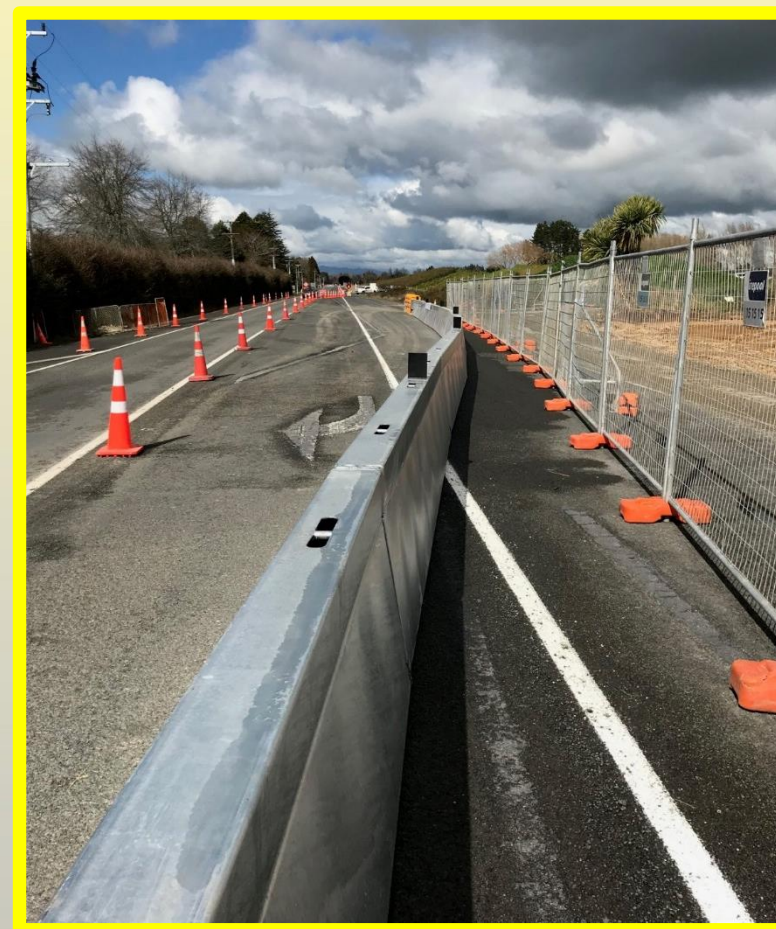
First HV2 Barrier installation in New Zealand
