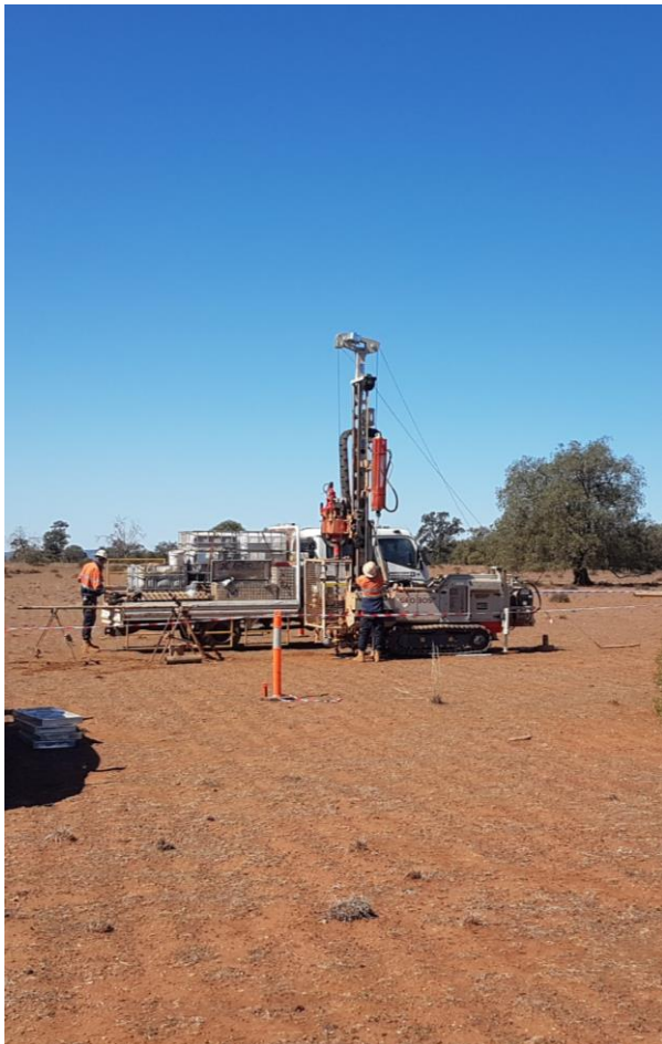
Geotechnical drilling on the proposed processing plant site
