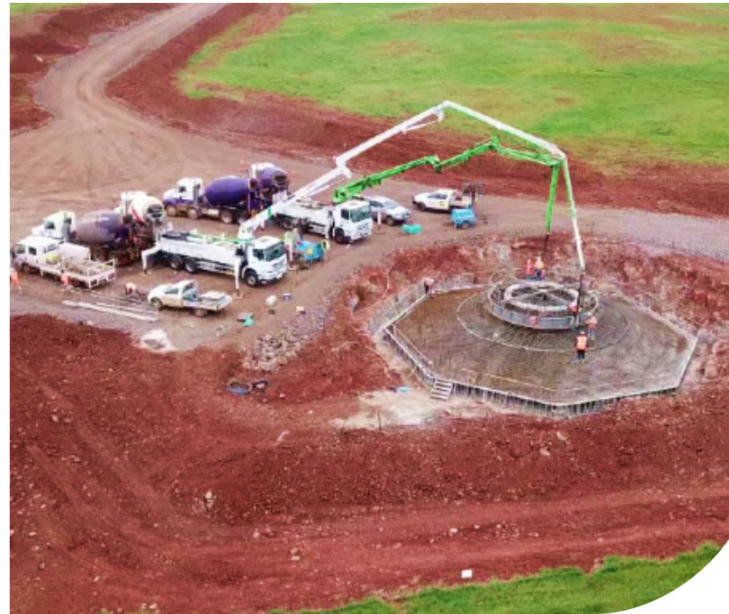
Wind turbine foundation being poured
