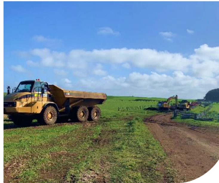
Civil works equipment onsite, establishing access
