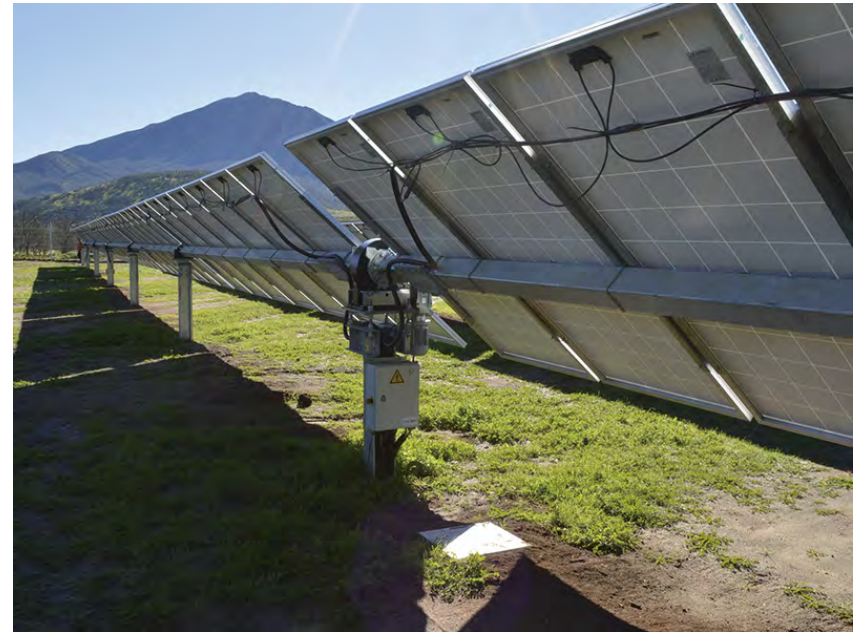
Example of Trina PV Modules on tracking system www.trinasolar.com
