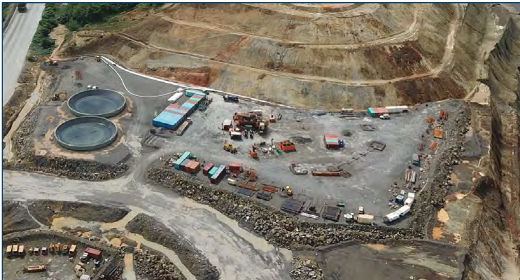
Directional drilling and cold water injection pad
