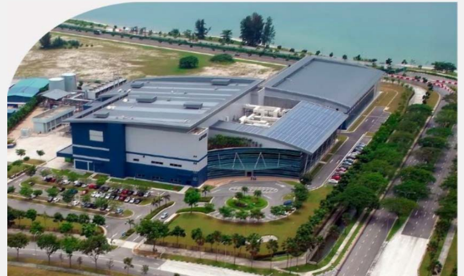
Lonza contract manufacturing facility in Singapore
