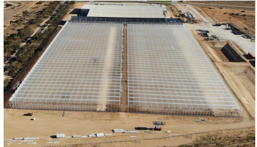
Image of Mildura facility – construction well underway
