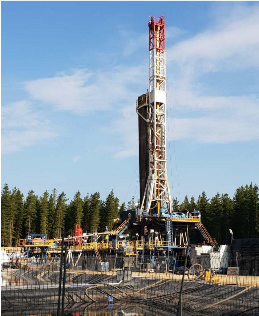
Easternwell Rig 106, on-site
