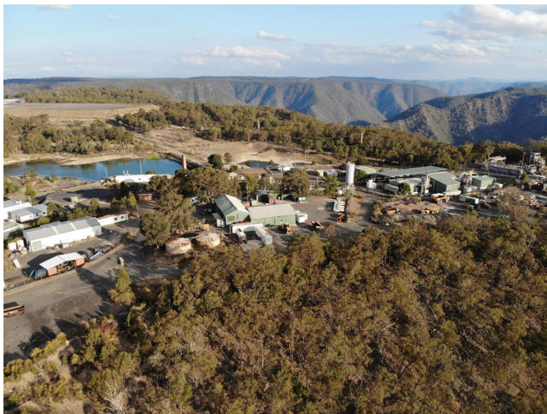
Figure 4 Hillgrove Gold Mine showing processing infrastructure and layout
