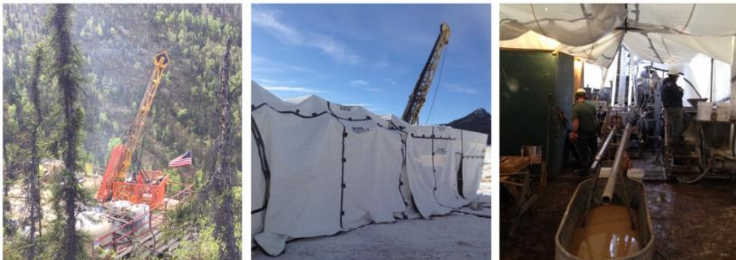
Figure 1. Ruen Drilling operating at projects across Alaska
