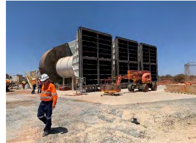
Installation of surface fans at Gwalia
