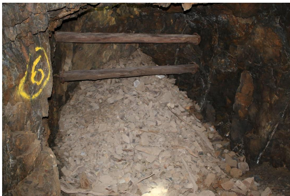
Figure 8 Draw Point 3 (DP3) 1700 Level
