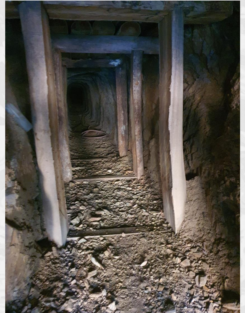
Refurbished Adit at Snowstorm, where 3D structural mapping has begun
