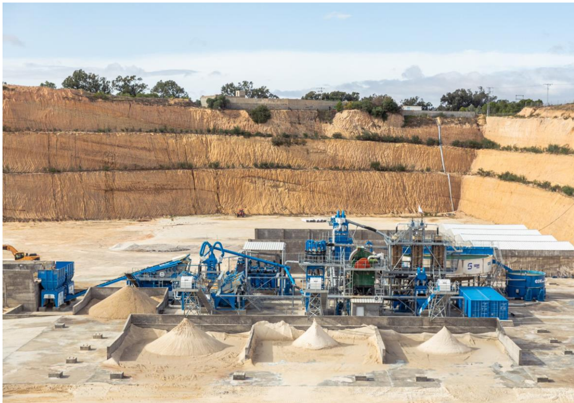
Figure 1: 200tph silica sand wash plant installed for SOMEVAM (Sebri Group) in Tunisia
