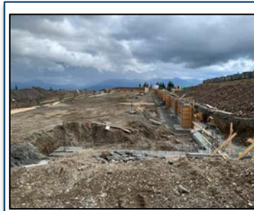
Permanent long term core processing facility under construction
