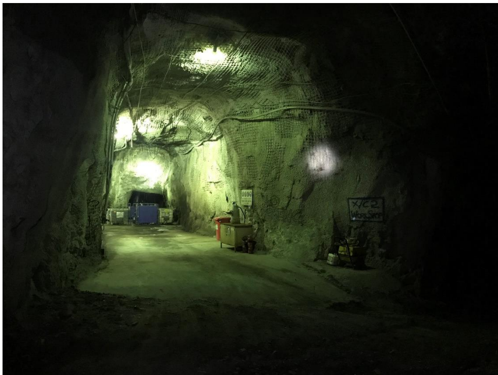
Figure 8 Metz Mining Centre UG Maintenance Workshop
