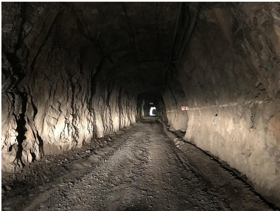
Figure 6 Metz Mining Centre Decline
