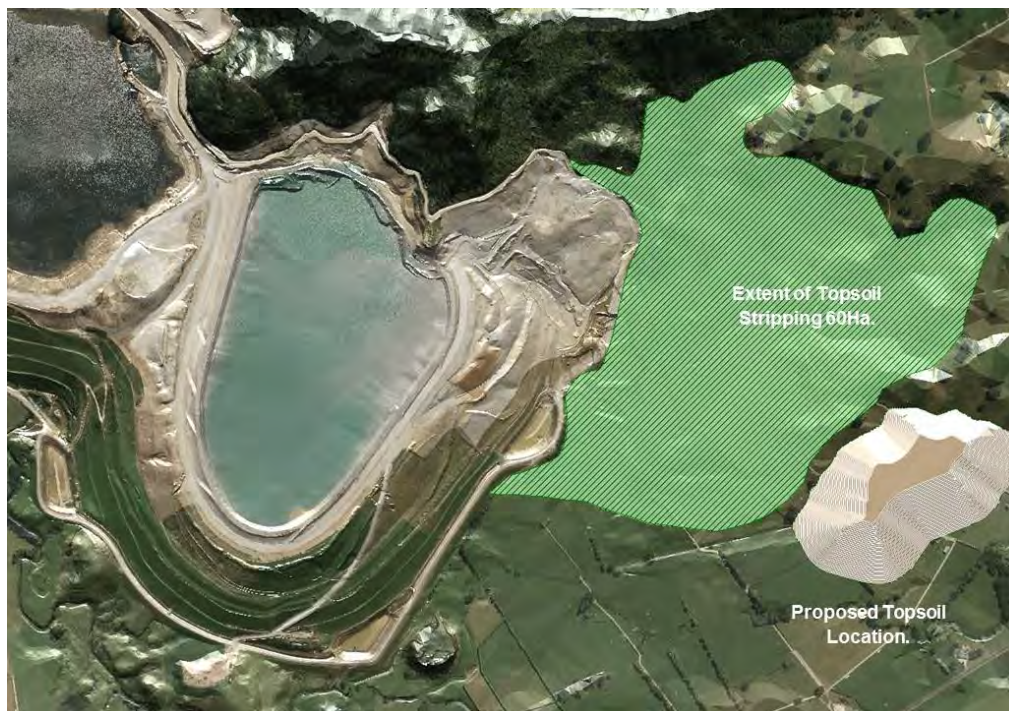
Figure 18-4: Preparatory Works for TSF3
