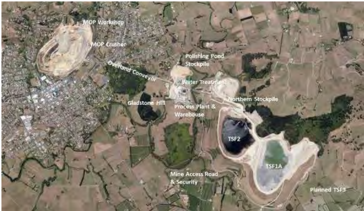
Figure 18-1: Waihi Existing Infrastructure
