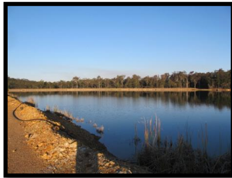
Mt Carrington Tailings Storage Facility
