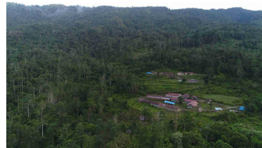
Awak Mas Camp and Core Storage facility
