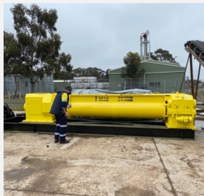
Ashley Moore, Group Chief Engineer, inspecting equipment as it arrives on site.
