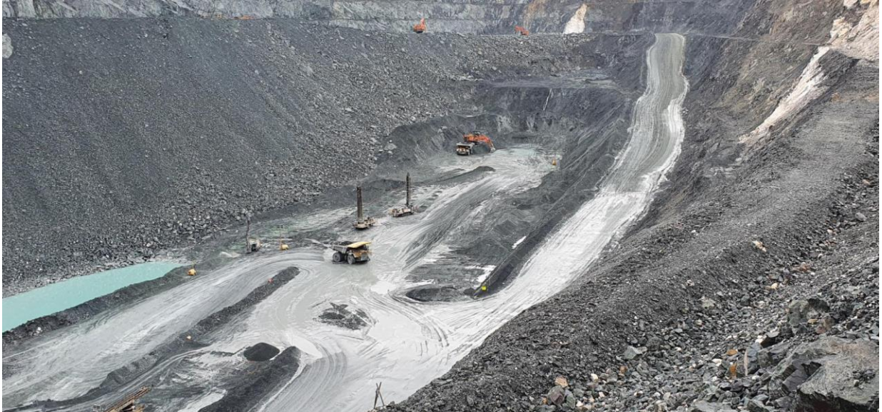
Mining in North Pit, Savage River
