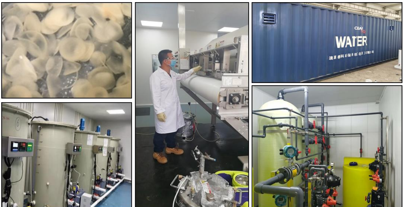
Clean TeQ's BIONEX manufacturing and pilot plant in Tianjin
