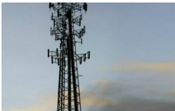
Mobile Phone Tower Crown Castle International Corp (US) Mkt Cap (July 2020): A$98 billion
