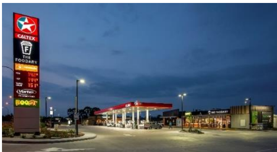
Brisbane Airport Link Service Centre
