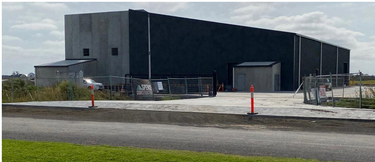
Image: Completed infant formula building (roof to be installed and some final works to be completed once plant installation has been completed)
