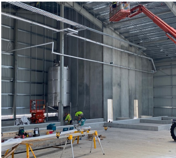
Images: Installation of liquid mixing tanks and internal fit out of the production facility
