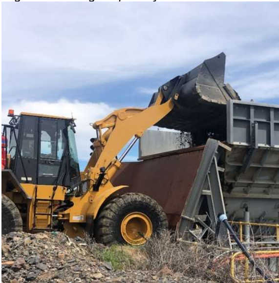
Figure 7 Feeding the primary crusher
