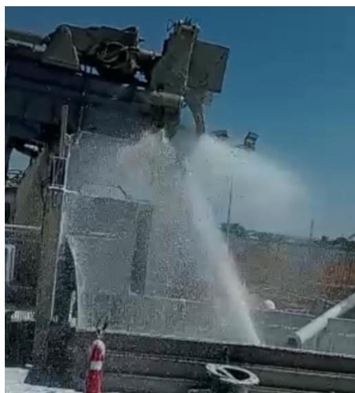
Image 1: P007 gas flowing to surface
