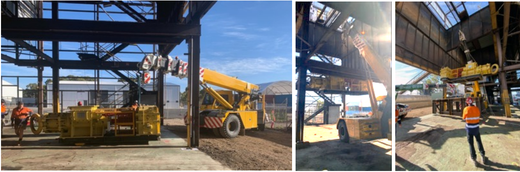
Above: Extruder being lifted on to its structural support.
