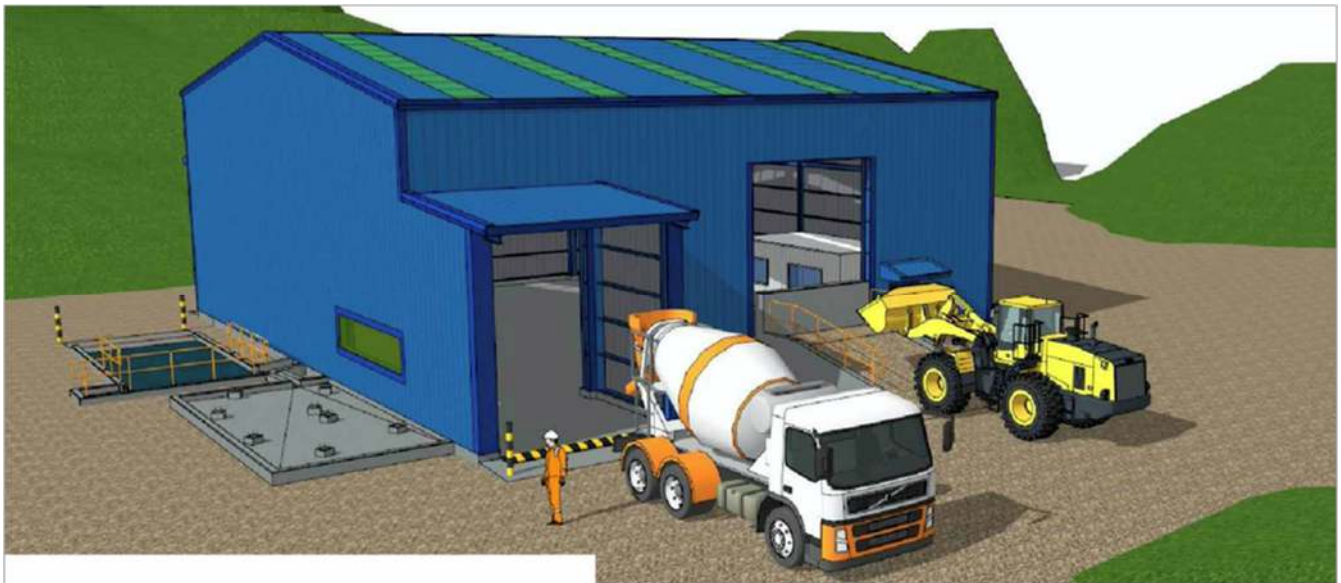
Figure 16-27: Dry Mix Cement Backfill Plant
