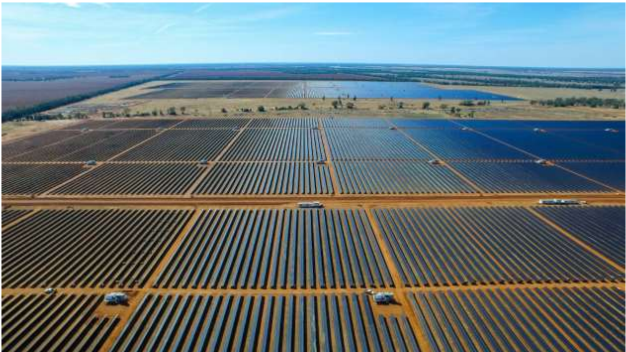
AGL's Nyngan Solar Farm, Central New South Wales
