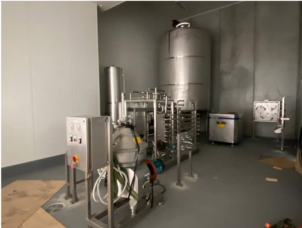
Image: Equipment being installed at the Infant Formula Plant
