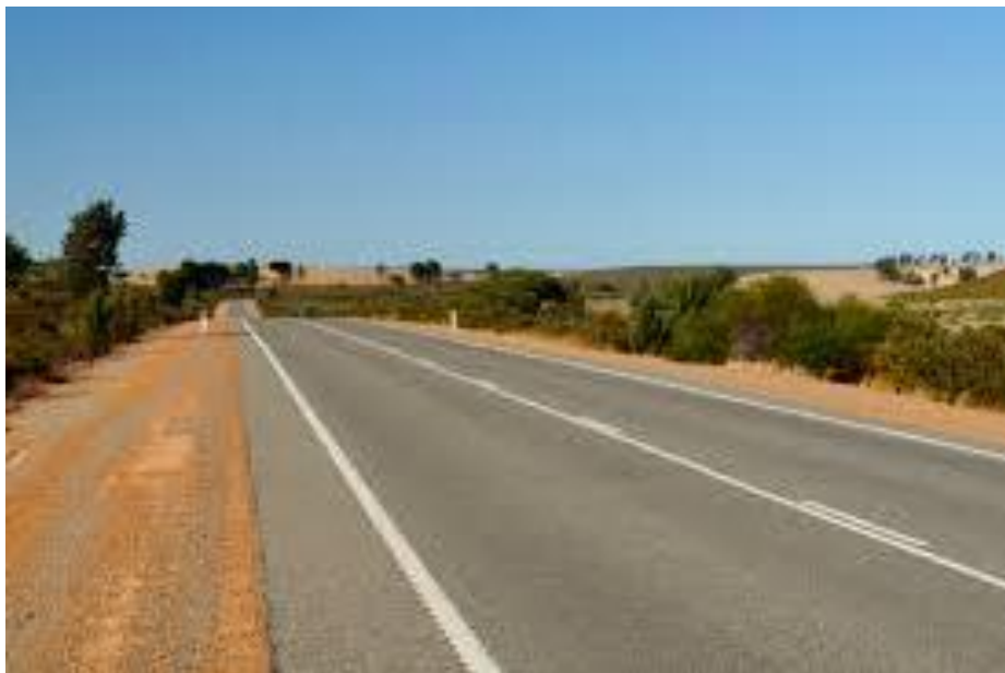
Brand Highway Proximal to Beharra
