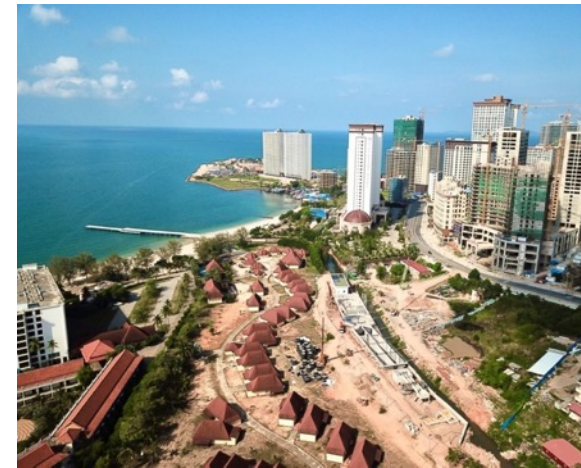
Construction site on April 2, 2021; commissioning in May 2021
