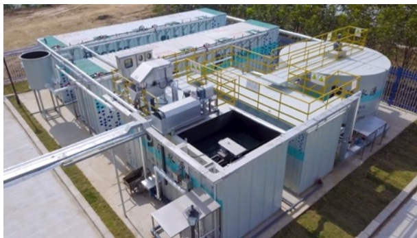
Rural Aspiral plant, Luoyang, Henan province
