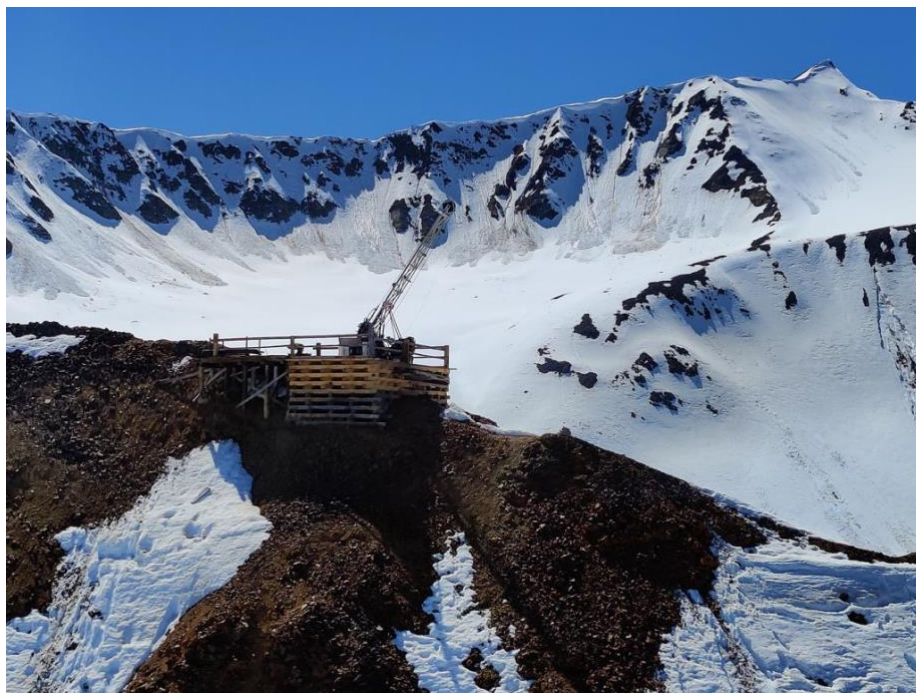
Figures 3 and 4: Drill Mobilised to First Hole Location at RPM
