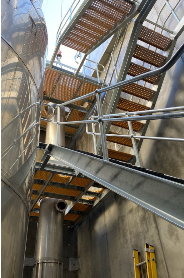
Image: Installation of stairs and platforms around evaporator
