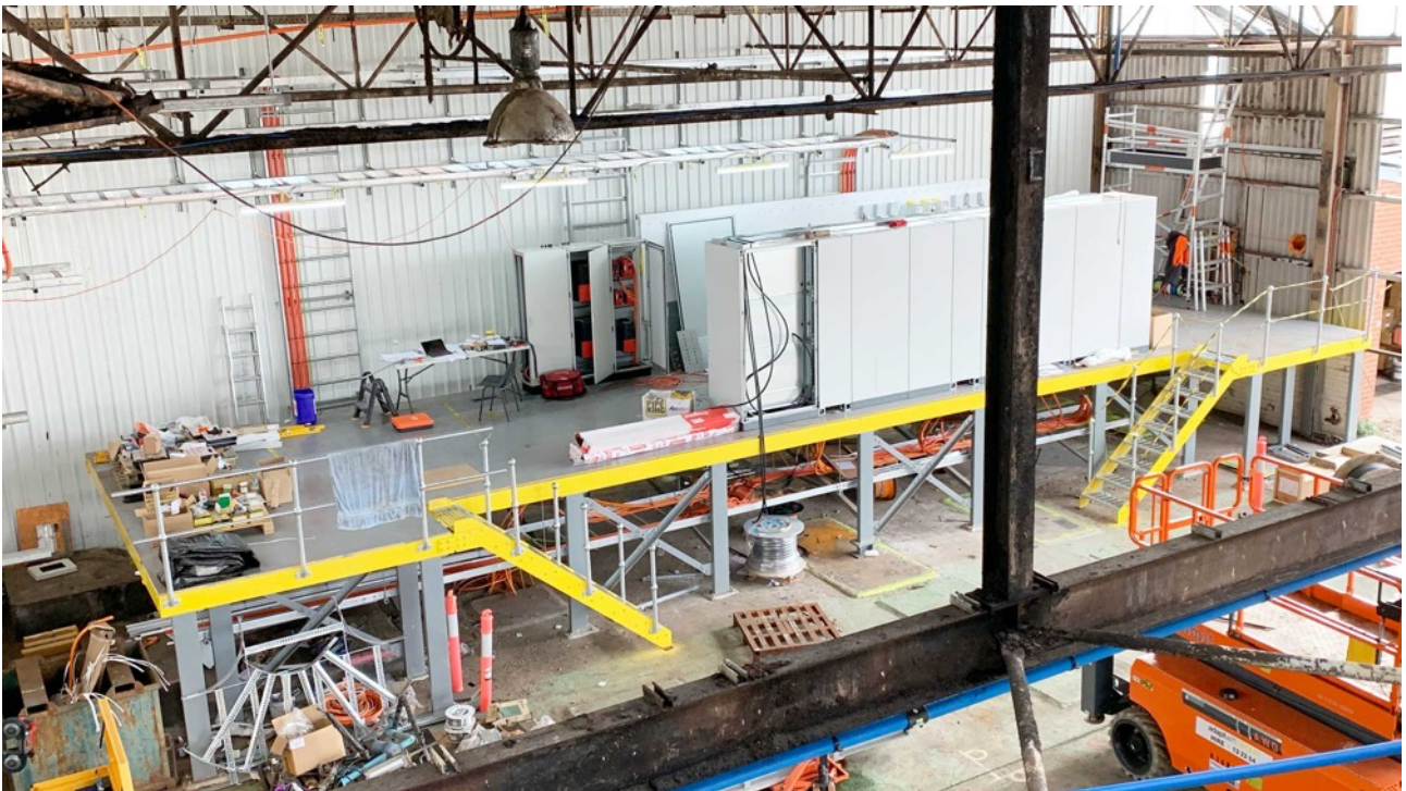
Above: arrival and installation of MCC (motor control centre) cabinets, which will house the electrical controls for the various functions of the plant.
