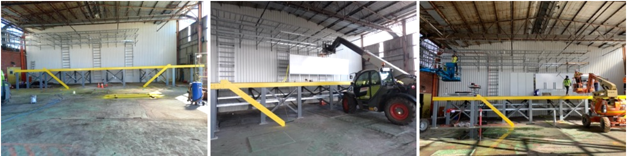
Above: (left) MCC floor installed and painted, (centre) installation of mounting wall for motor variable speed drives, (right) pull through of cables from mains to MCC.
