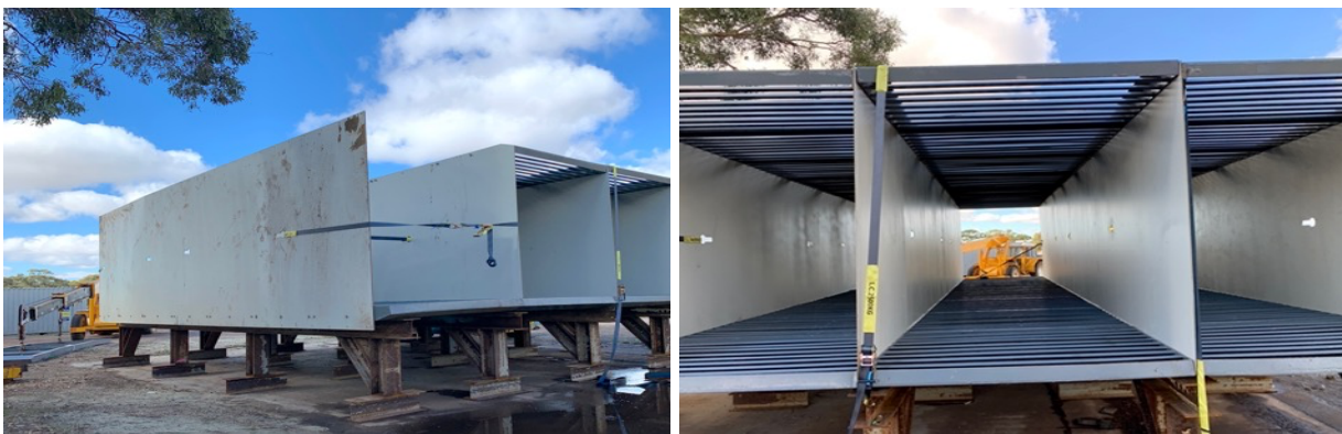
Above: assembly of the updated design for the internal walls of the packed bed dryer.
