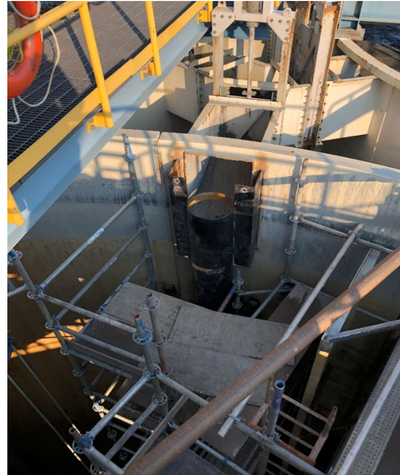
Downcomer installation in leach tanks at Touquoy processing plant
