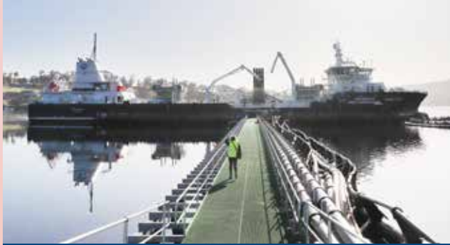
'FISH OUT PIPES' TO RONJA STORM
