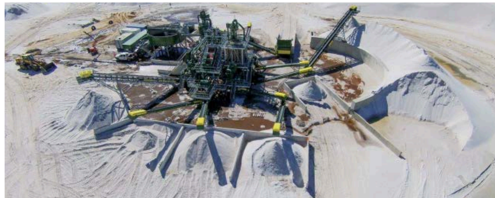
Typical sand plant showing various product streams being produced
