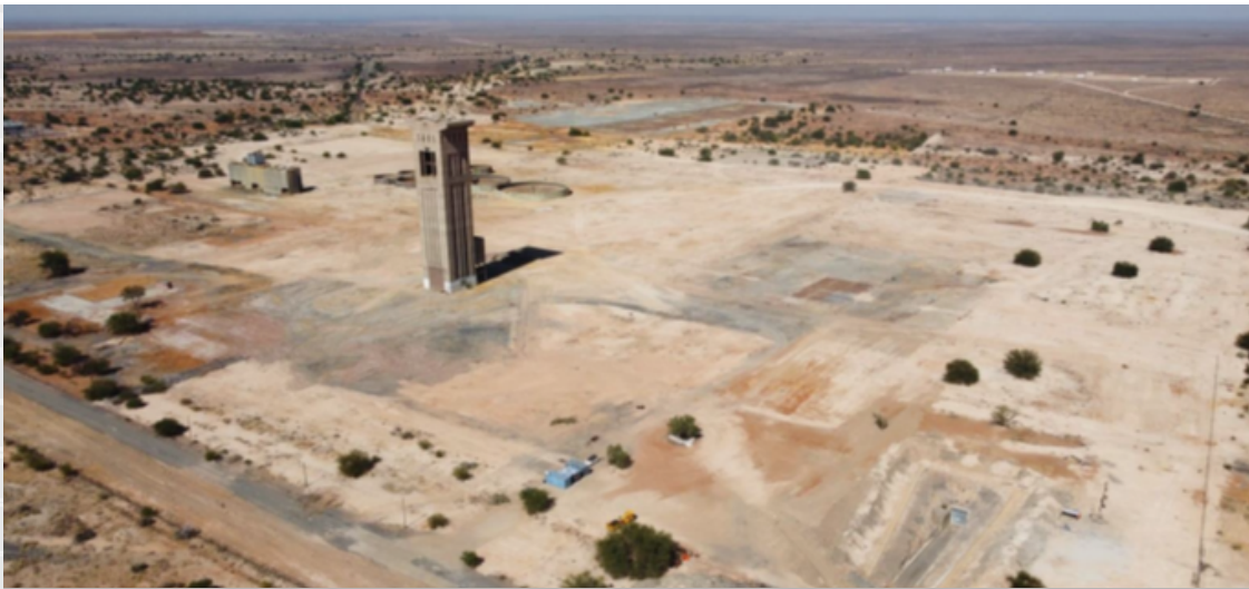
FIGURE 4: HUTCHINGS SHAFT AREA AFTER SURFACE AREA CLEAN-UP.
