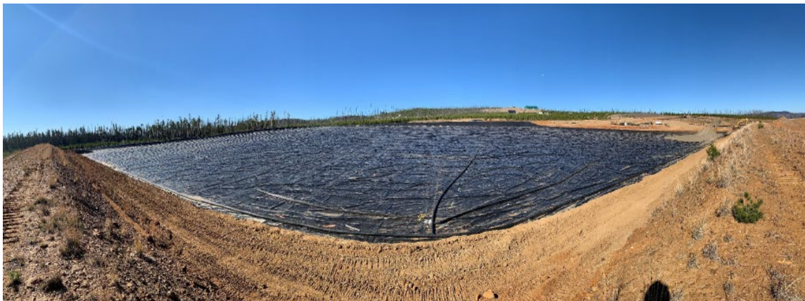
Tailings Waste Storage Facility: View looking west. 8-inch drain line installed, continuing to install additional piping. Entry ramp to the right has started and will be the main conduit for bringing in drainage rock.
