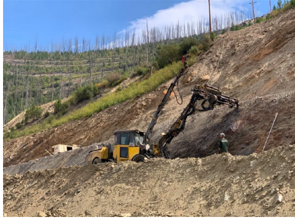
LEFT: View of bolter installing MAI grout bolts. SMD is currently installing the bolts. Once bolts are installed grout (Portland Type 2) cement will be inserted through the grout bolts.
