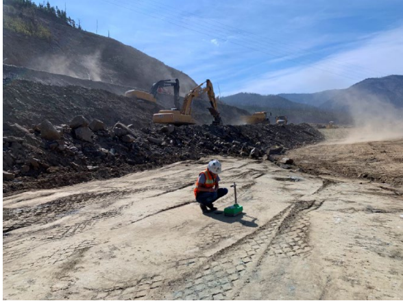
LEFT: View looking west along portal bench raise. Western Materials conducting compaction tests. Compaction results about 95-98%
